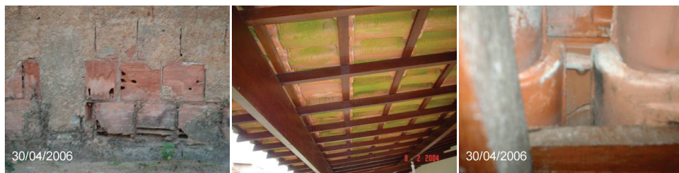
Fig. 1. Fast degradation of masonry and tiles
