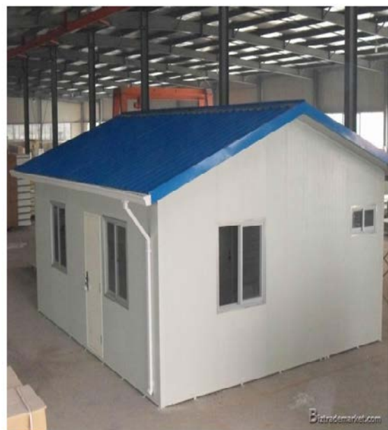
Figure1. Basic prefabricated house
