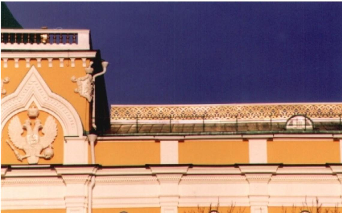
Fig. 6 Decorative grating for the reconstructed roof of the Great Kremlin Palace in Moscow. The individual elements (laser patterned and TiN coated 1×2 m stainless steelstrips) are visible
