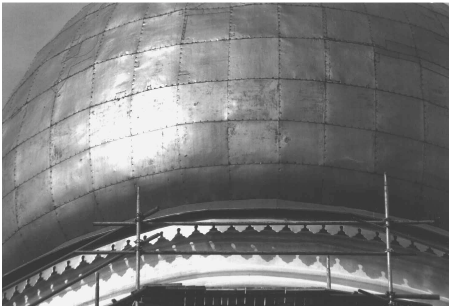
Fig. 8. Failure of conventional gold coating (roof of Holy Mary Cathedral in Kremlin, about 6 years after coating with thin gold foils)
