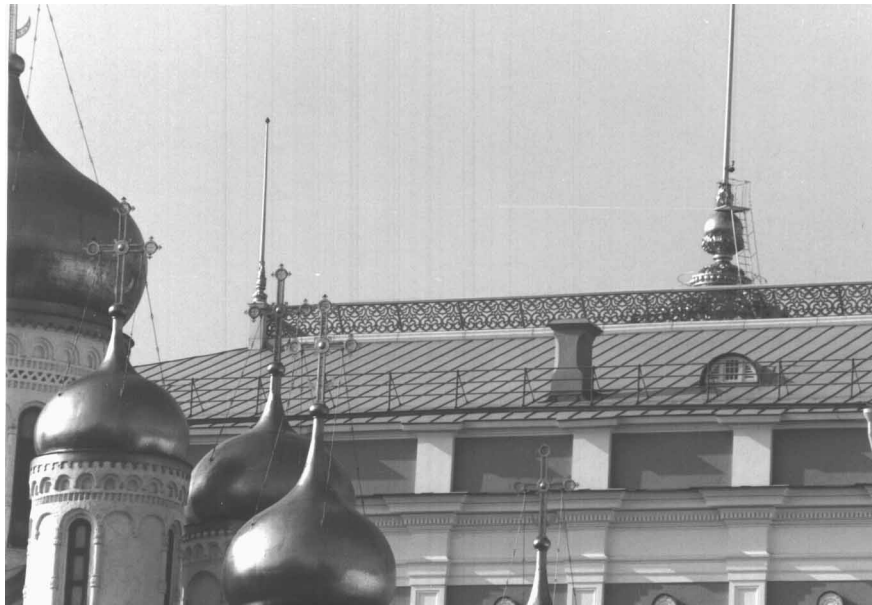
Fig. 6. Decorative grating for the reconstructed roof of the Great Kremlin Palace in Moscow. The individual elements (laser patterned and TiN coated 1×2 m stainless steelstrips) are visible. In the foreground the domes can be seen freshly coated with thin gold foils (using the conventional method)
